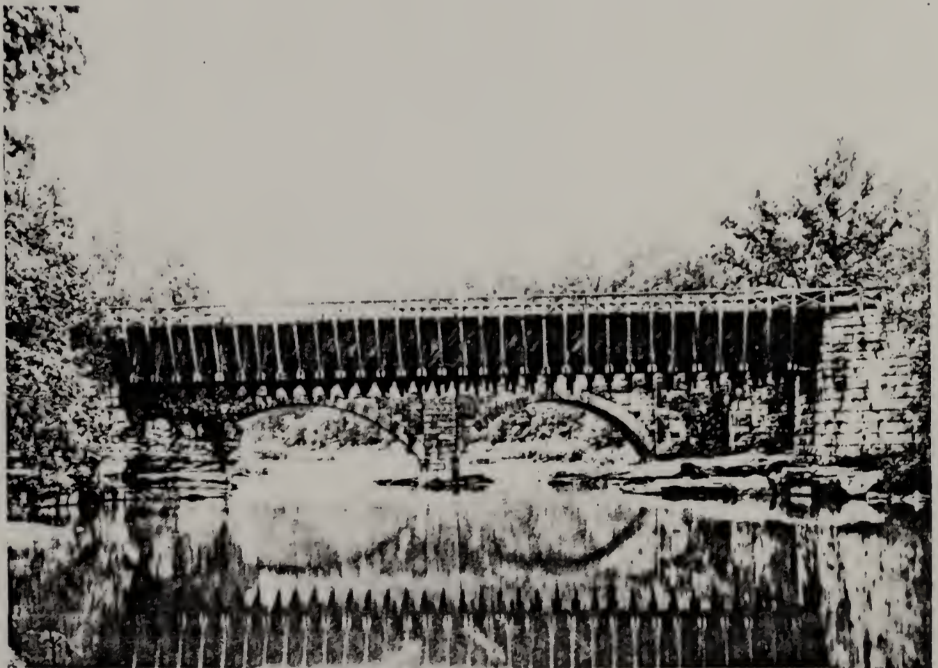
The Suspension Aqueduct at High Falls, Pennsylvania, Built by John A. Roebling and Employing the Wire Rope Suspension Principle
